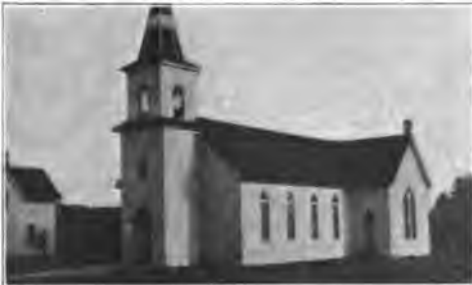
Kirke, 1880, $2,450. Skolehus 1, 1863. Skolehus 2, 1870, $1,500. Prestehus, 1892, $5,000. Land, 4 lotter, $5,000.
